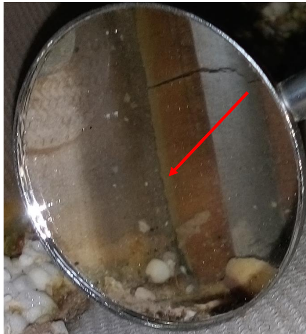
Fig. 5: Loosening of the rib from the spar
