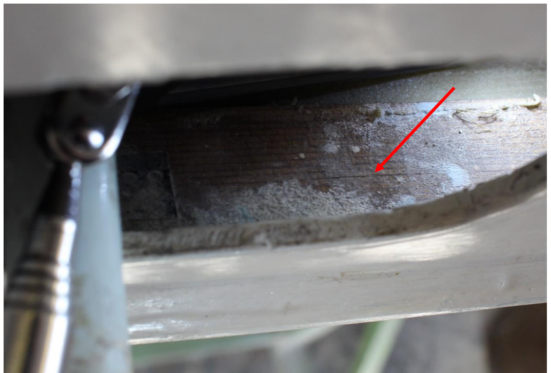
Fig. 3: Cracks parallel to the root rib plane
