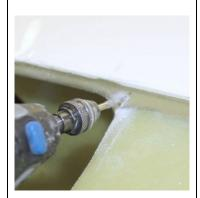
Remove the crack by milling (as v-shaped as possible) until the root of the crack.
